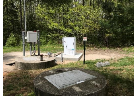
Progress on the Admiral's Way pump station.
