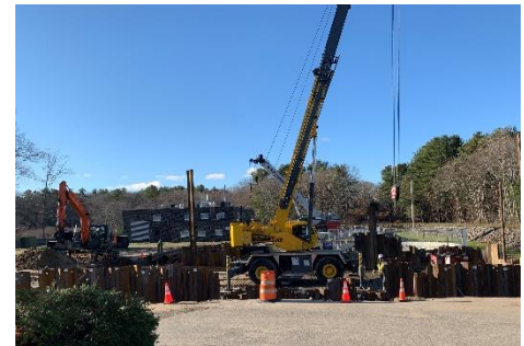
Construction has begun
