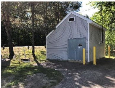
Cat Mousam Road Pump Station
